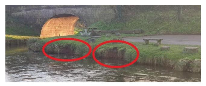
After looking at various possible solutions, it was decided that recycled plastic piling would provide the most long-lasting and cost-effective for of bank protection at this busy location.
