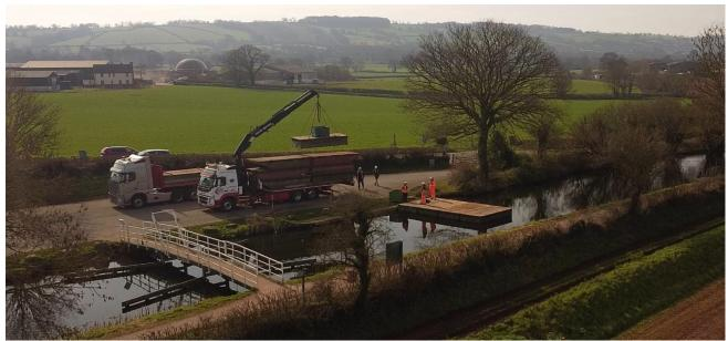
Once the pontoon was assembled, the excavator boarded and the weedboat was used to push the pontoon for half a mile to the far end of the section being dredged.
