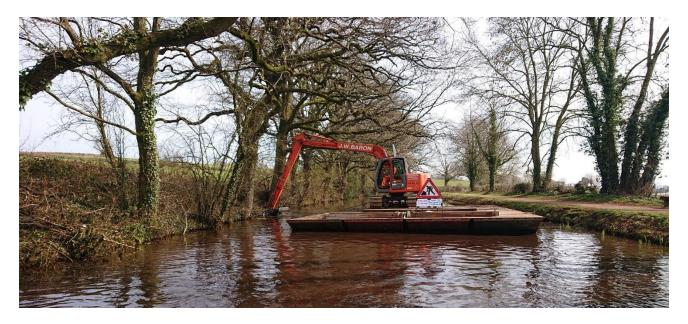
The contractor then spent five days dredging the section, with mud and debris being spread on the offside banks. The work should ensure that this section of canal remains navigable for many years until the next full-scale dredging programme takes place.
